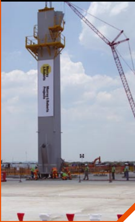
■ Setting of the first boiler house column at Medupi power station
