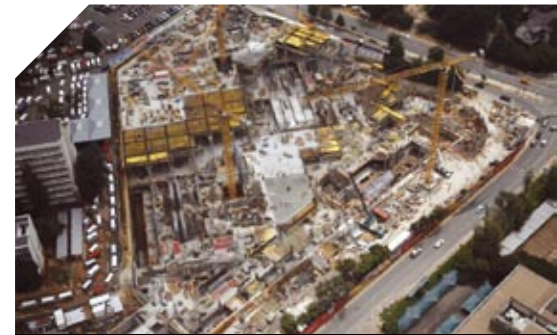
■ Sandton Station. View towards west – 28 January 2010
