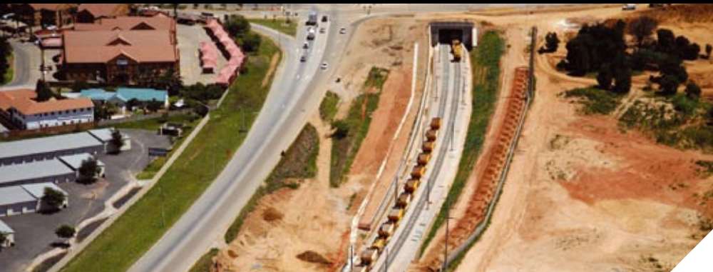
■ Depot to Midrand Station. View towards the north – 18 December 2009
